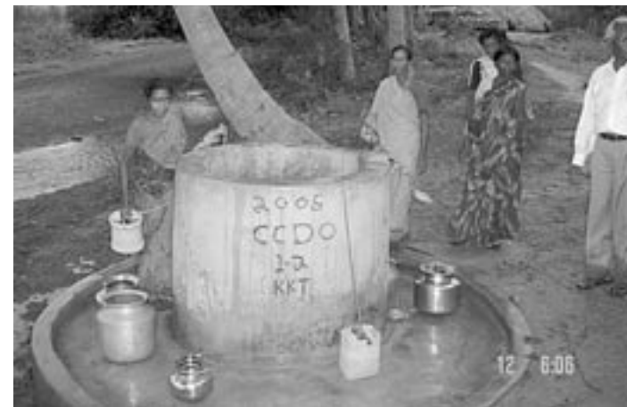
The style of well depended on the local terrain. All wells have concrete pads and runoffs to prevent contamination.
